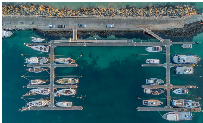
Apollo Bay Harbour Redevelopment
