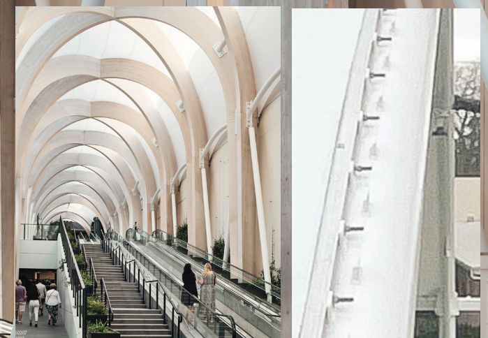
View of Roof Inside Open Air Access Link
