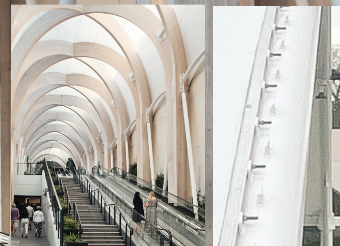
View of Roof Inside Open Air Access Link
